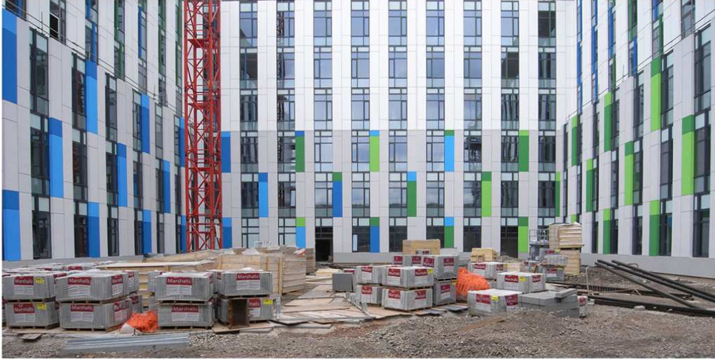
Metal and Render - during construction
