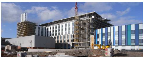
'DTC Block - Glass spandrel panels and metal fins - On site during construction' King's Mill Hospital. Collaboration with Swanke Hayden Connell Architects and SKANSKA 2006
